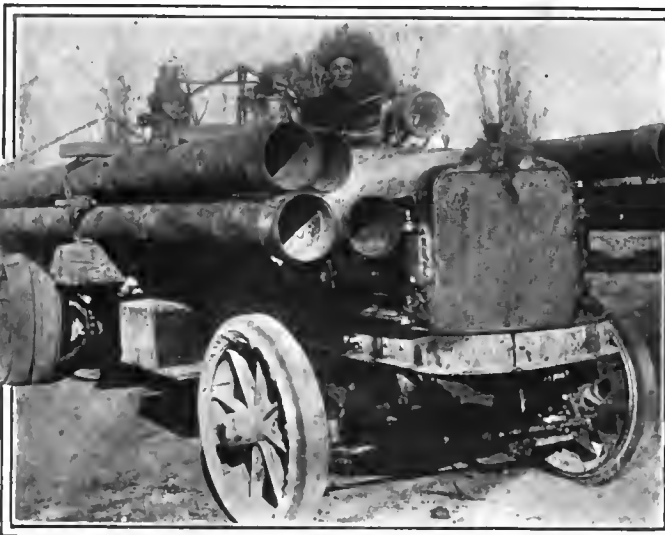
How the pipes were carried, ready to drop at the roadside
